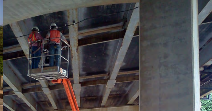
Under: PM Road closure
