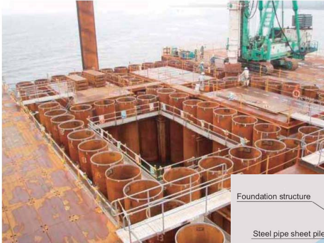
Photo 2 Steel pipe sheet pile foundation
