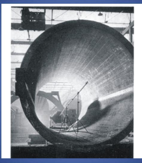
An iridium-192 source in use for the non-destructive testing of a welded steel shell at the works of G. A. Harvey & Go. (London) Ltd.
