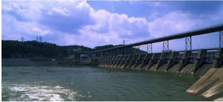
Watts Bar Dam Construction 1939 - 1942. 112 feet high and stretches 2,960 feet across the Tennessee River.
